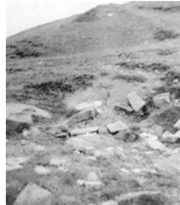
Plate 9: The displaced pipe, as we found it.
